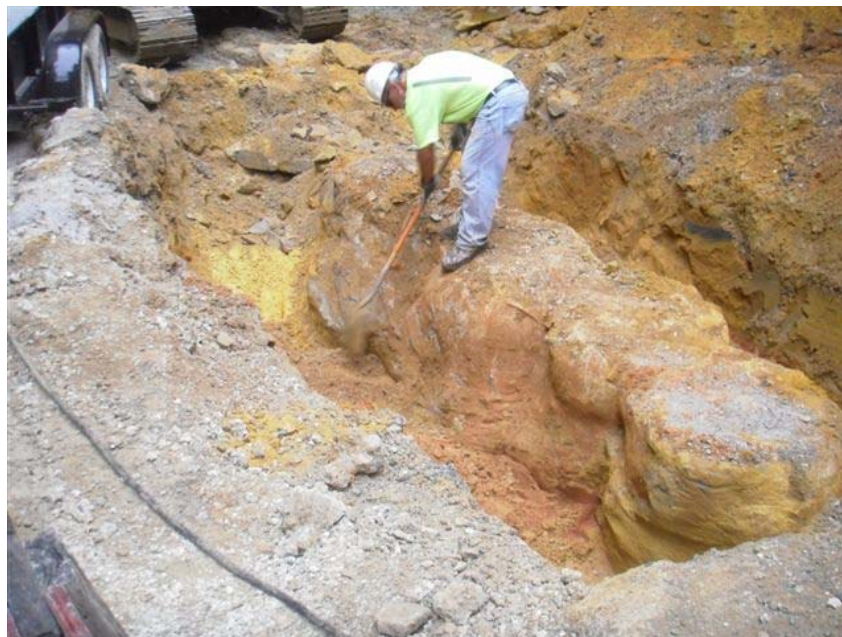
Photograph 4. Exposed miniJET® columns showing average 40-inch diameter.
