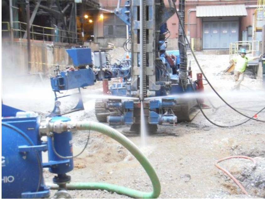
Photograph 3. MiniJET ® system being prepared for insertion.
